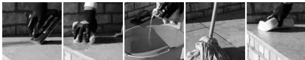
PIC 1. Fill joint with grout.
